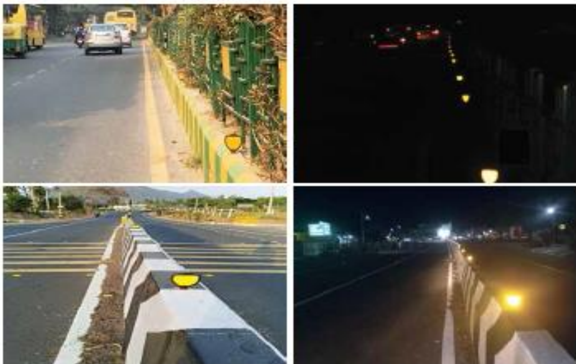
Fig. 8 Typical Illustration of Utility of Flexible Median Markers during Day and Night Time
